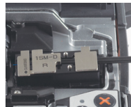
Drop cable splicing with fiber holder system
